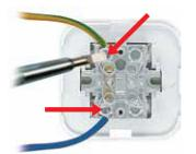
3 Place the connections and tighten the screws
