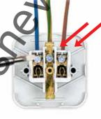
2 Place the connections and tighten the screws
