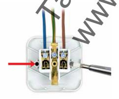
(3) Mount to the wall with fixation screws
