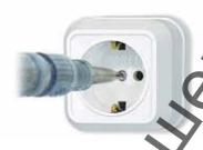
1 Remove the cover with screwdrive
